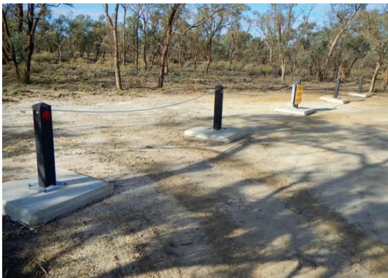
Karadoc bollard installation works - using bollards secured into precast concrete slab ensures no ground disturbance is required for culturally sensitive areas.
