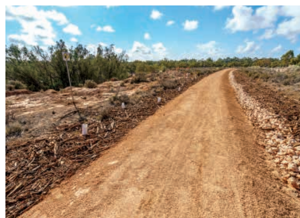
Completed walking track with swale drainage at Merbein Common.
