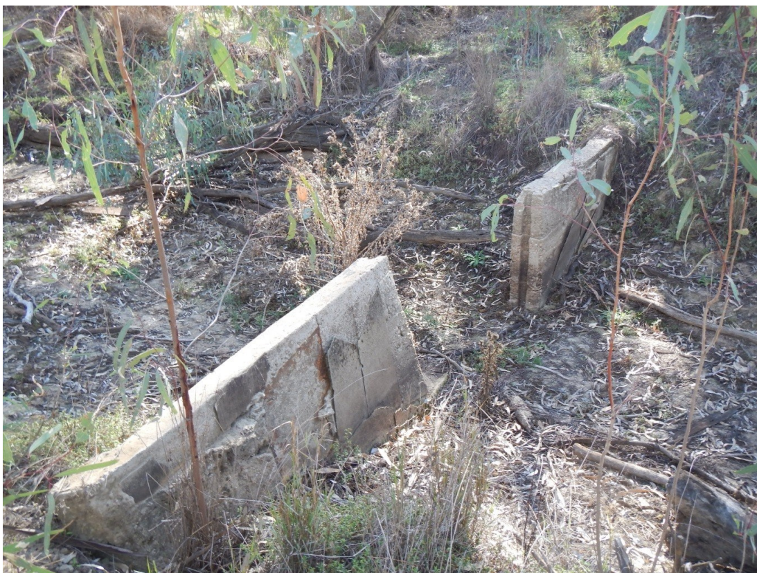
Figure 18. Photograph taken of a regulator structure in disrepair, this structure is located on the creek inlet to Central Fishers Lagoon
