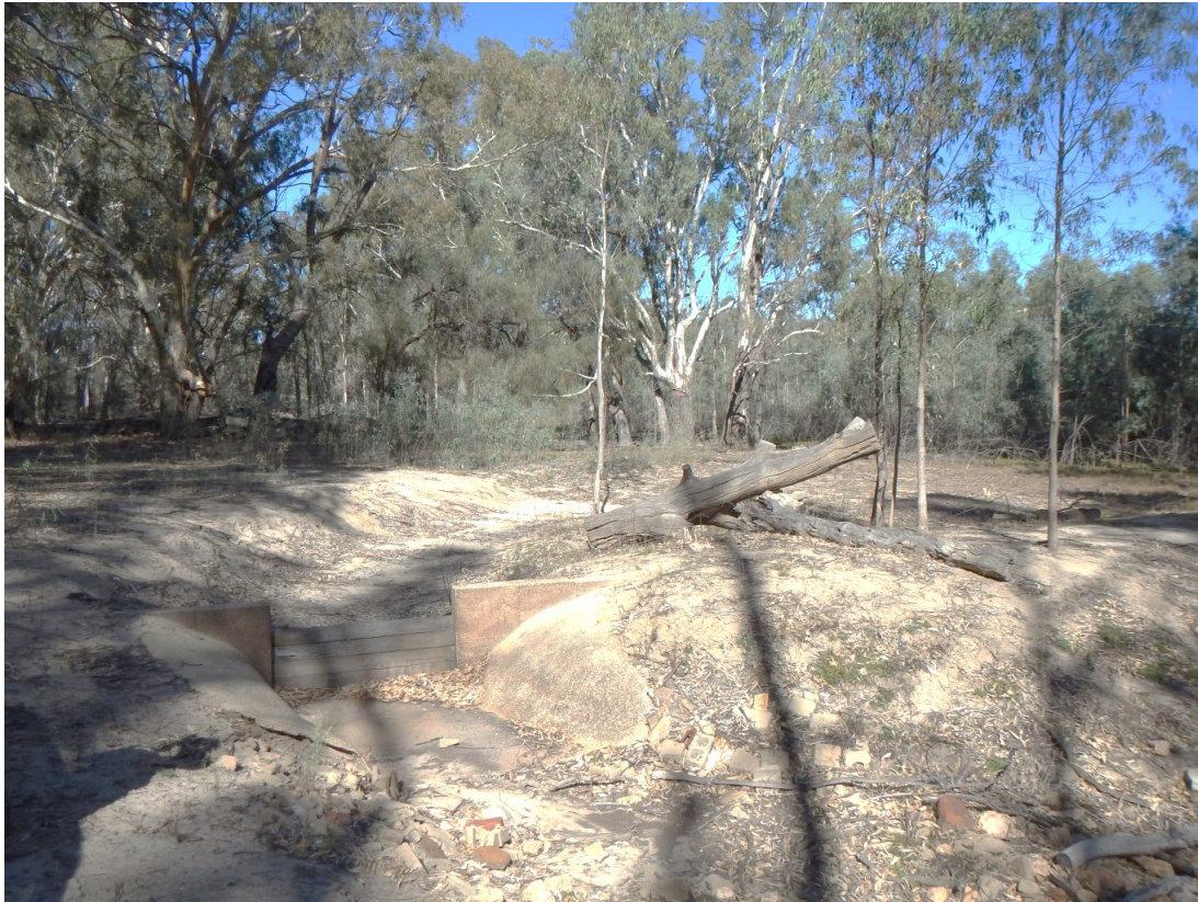
Figure 17. Photograph of a regulator structure still in use near the western end of Fishers Lagoon West
