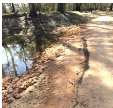
Figure 7. Levee constructed for delivery of environmental water to Bridge Creek
