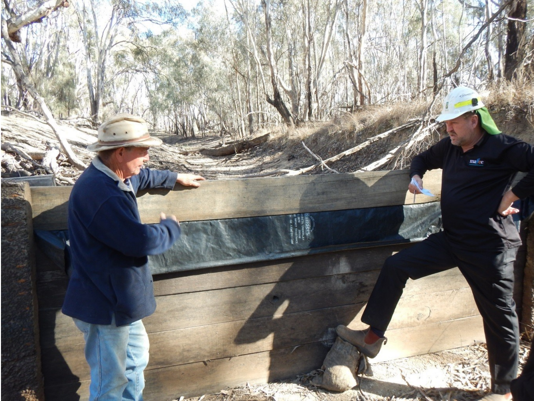
Figure 19. Photograph taken of a regulator structure not in use near the eastern end of Fishers Lagoon West.
