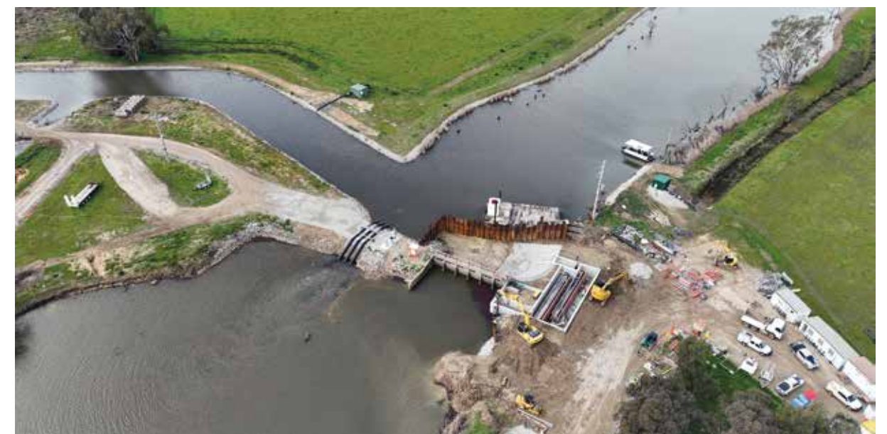
Work being undertaken on the construction of the Taylor’s Creek fishway, connecting 1,000 kilometres of waterways for native fish.
