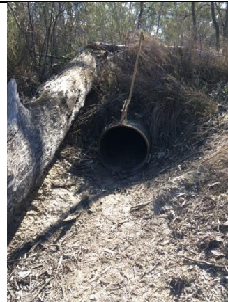
The upstream end of the pipe culvert at the cutting at Impediment 5. Evidence exists of past ability to close off the culvert.
