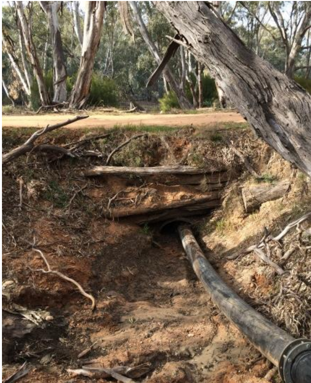
Figure 16 - Pump Site C and Impediment Site 22. Pipe shown is for delivery of environmental water, delivered through the existing culvert.
